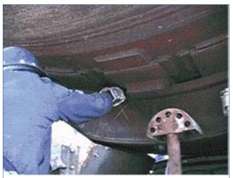
Figure 5. An operator inserts a lube bar between the tyre and the shell.
